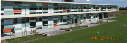
Solar collectors on the Administration block at Papamoa High school
