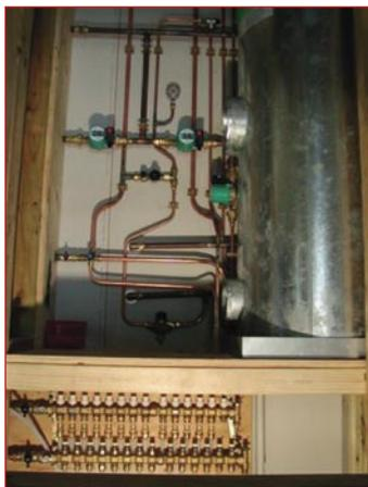
Figure 5: Solar heated cylinder with heat pump backup heating for underfloor heating system
