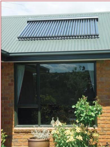
Figure 3: An evacuated tube collector installation
